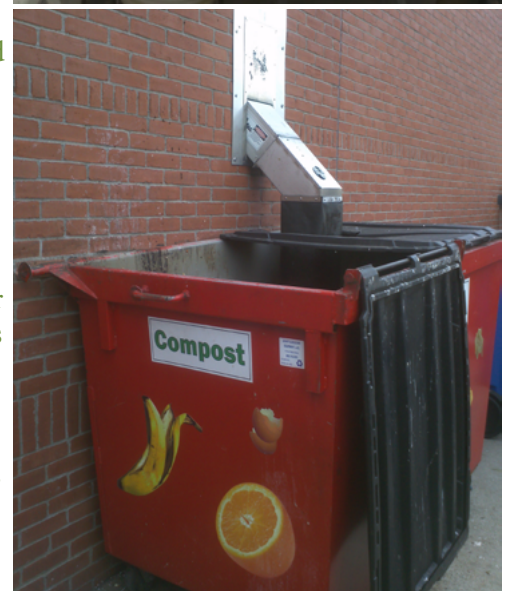
The Somat Centrifuge (top) directly feeds food scraps into a 2-yard container (above).
