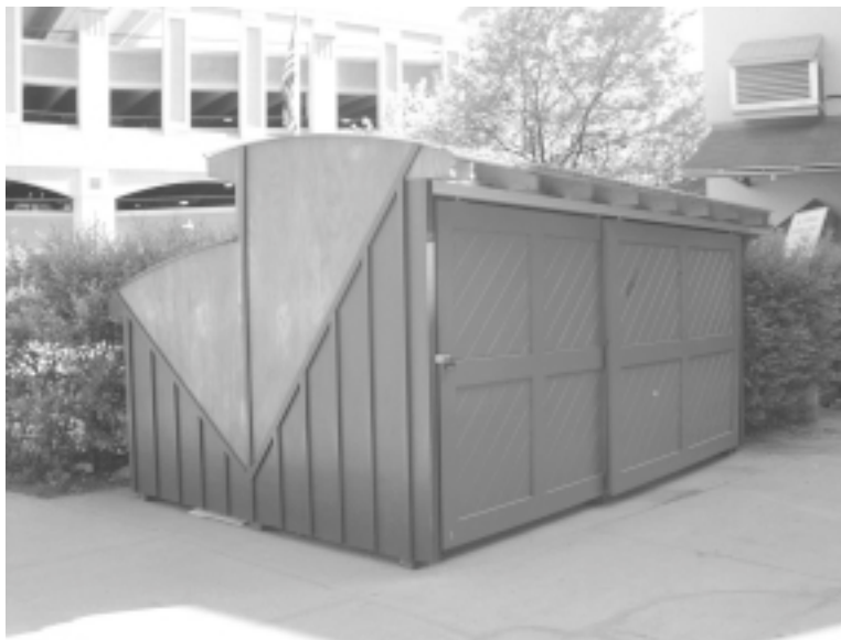
The shed serving Thornes Market in Northampton.
